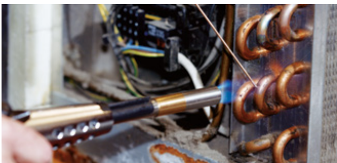
Brazing in refrigeration / air-conditioning technology
