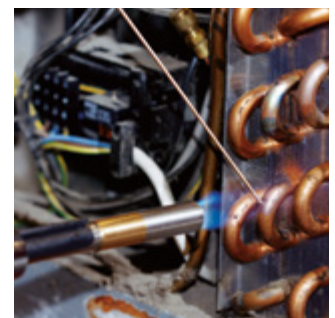
Brazing in refrigeration / air-conditioning technology
