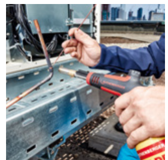
Brazing in refrigeration / air-conditioning technology
