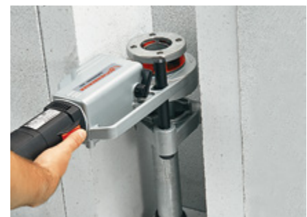
Work in confined spaces
