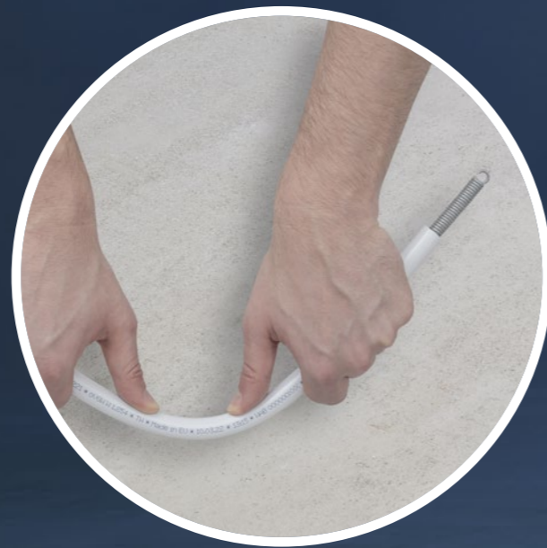
02 Pipe profiling with a spring.
