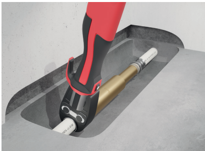
Fig. 30: Installation steps repair coupler.
